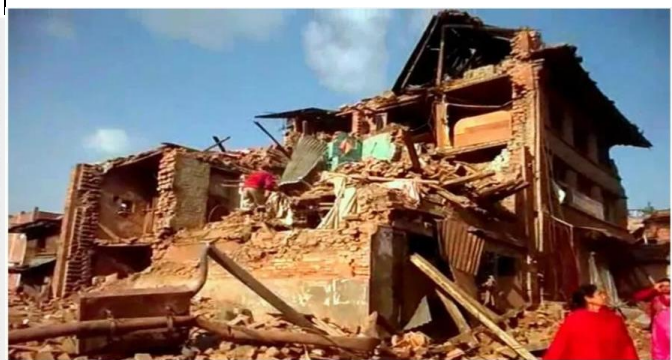
Building damaged during Earthquake of April 28, 2023 in Bajuar District
