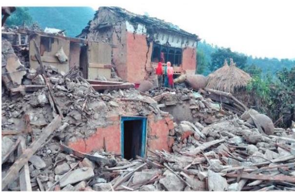
Building damaged during Earthquake of Nov 9, 2022, in Doti District
