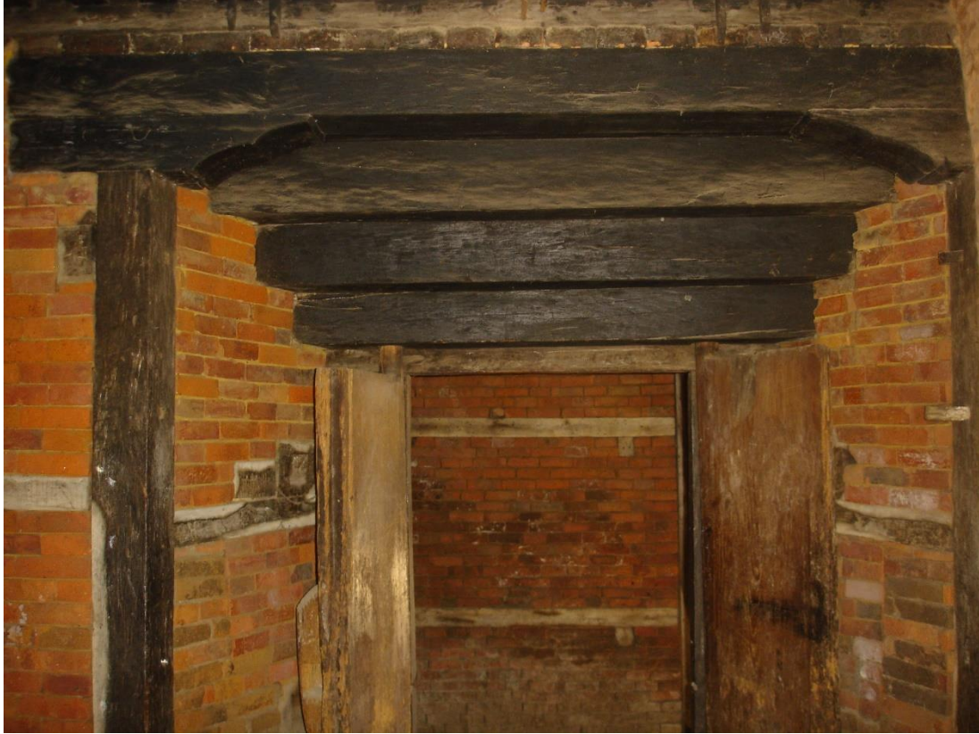
Figure 29. Double Framing in Door
