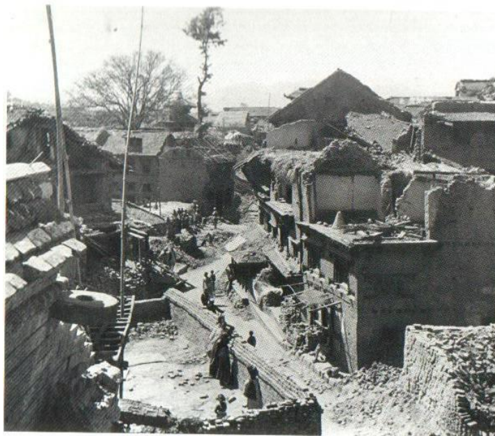
Figure 28. Photograph of a residential street in Lalitpur after the 1934 earthquake
