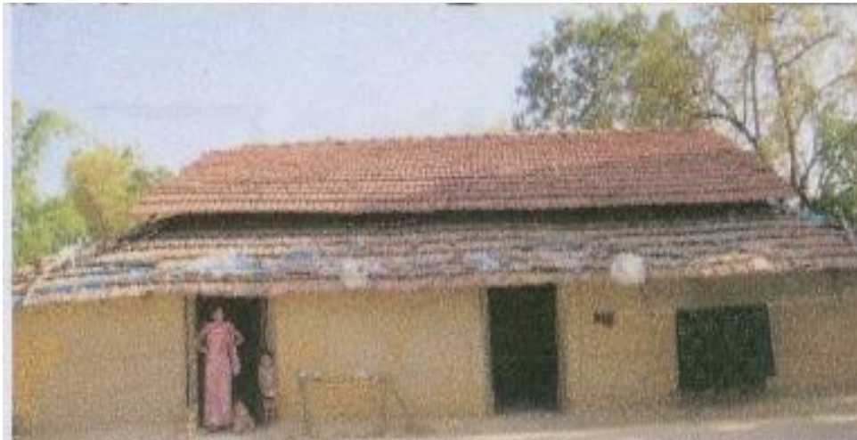
Figure 18. View of Dhangadi Residence of Terai
