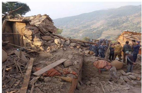
Building damaged during Earthquake of Nov 9, 2022, in Doti District
